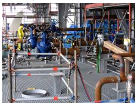
Figure 23: Example of Barricading of small opening
