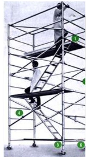
Figure 18: Mobile scaffold with integral staircases
