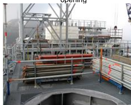
Figure 24: Example of Barricading of large opening
